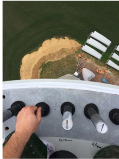
Filling the gap and force lock the connection between the tower segment and wind turbine machine.
