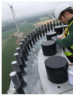
Filling the gap and force lock the connection between the tower segment and wind turbine machine.
