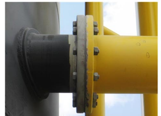
Filling the gap between ladder connection and tower segment
