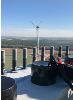
Filling the gap and force lock the connection between the tower segment and wind turbine machine.
